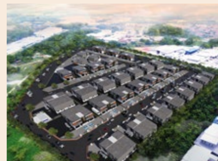
PARAMOUNT PALMERA Industrial park development
